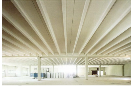
Figure 4.50: Plancher nervuré
