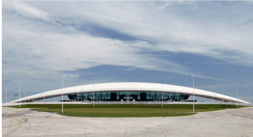
Figure 3.10: Façade principale du terminal
