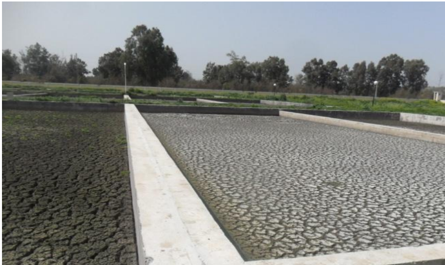
Figure III.8 : Lit de séchage (ONA.2013)
