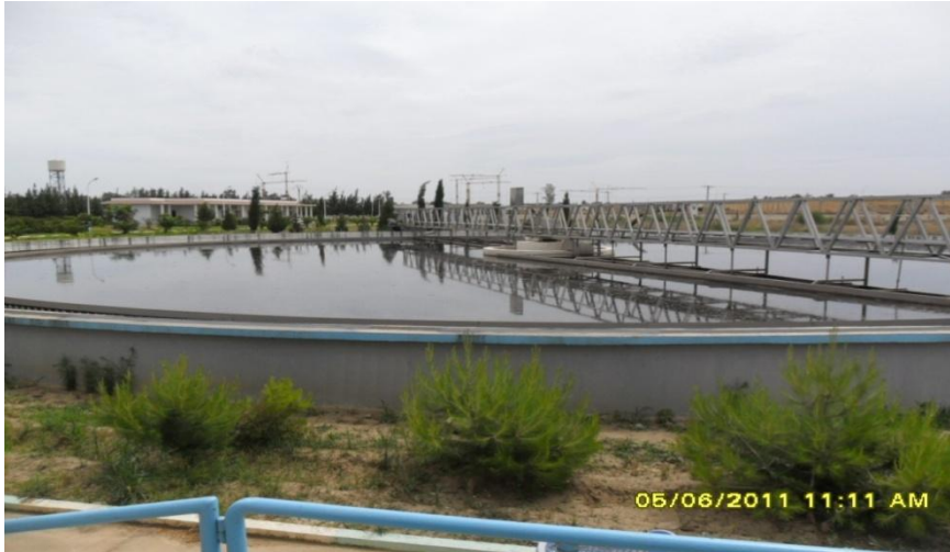
Figure III.6: du bassin de clarificateur (ONA.2011)
