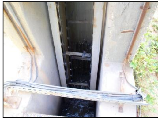
Figure III.5: Grille Automatique (22/05/2012)
