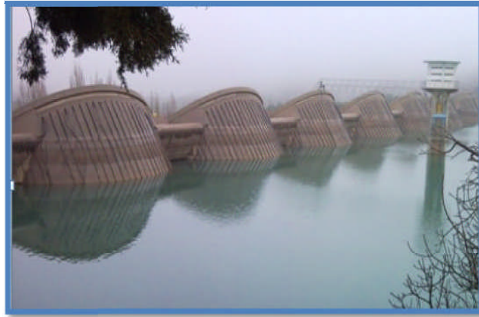
Figure 3.7 : Barrage Meffrouch (Photo Fellah H.S., 2009).
