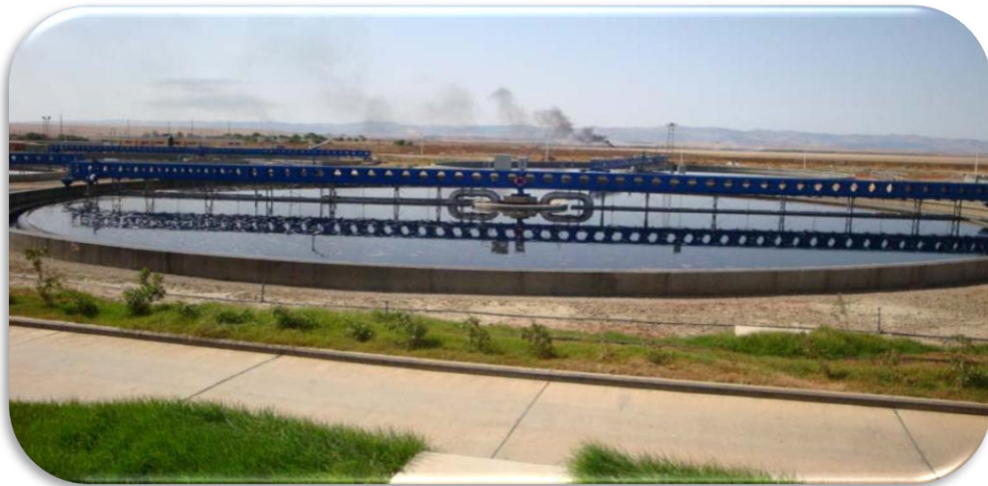
Figure III.6. Décantation secondaire
