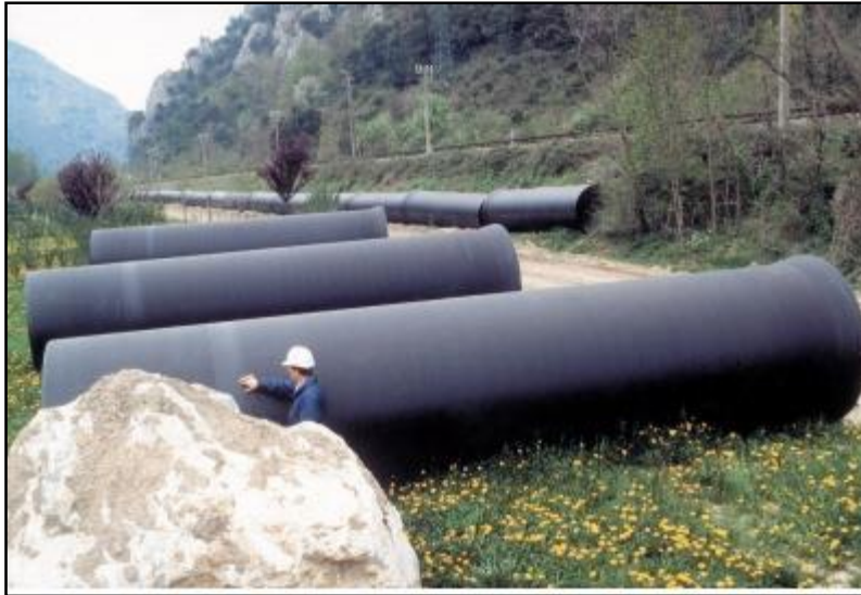
Figure I.4 : canalisation en fonte ductile. (Godart.H, 2008)
