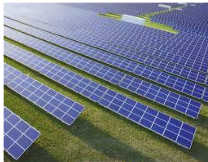
Figure (I.19) : Un champ photovoltaïque
