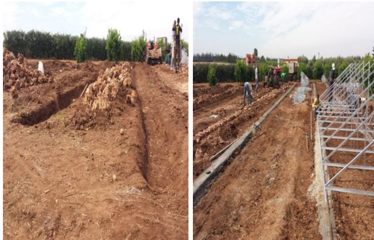
FIGURE III.1 – Implantation des socles
