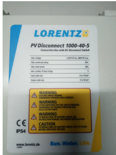
FIGURE 14 – PV Dissconnect
