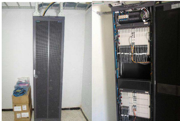
Figure III.29 : Armoire MSAN
