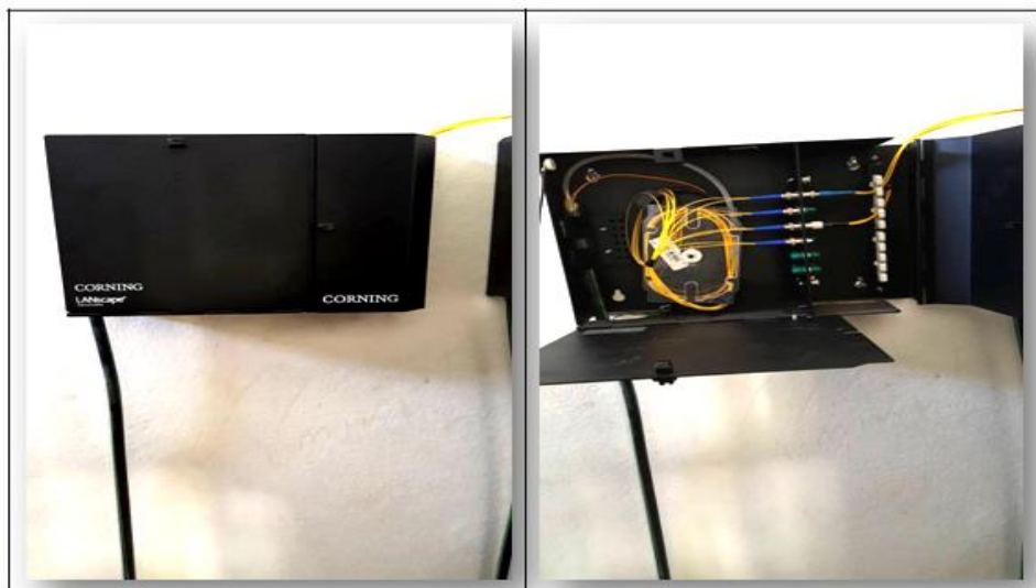
Figure III.11 : coffret optique mural
