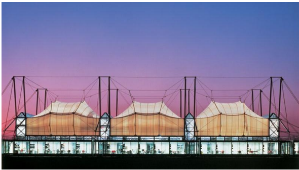
Figure 23: Vue de façade principale.
