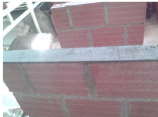
**Figure 3.23 :** Le surfaçage horizontal.
