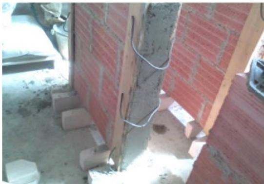
**Figure 3.22:** Le surfaçage vertical
