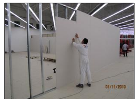
Figure 96: cloisons en Placoplatre
