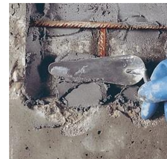
Figure 4.20 : Application du mortier
