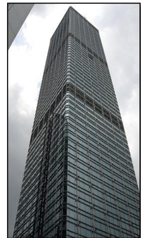
Fig.45 : Cheung Kong Centre, Hong Kong
