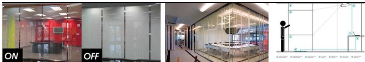
Fig. 203: principe des cloisons interactives
