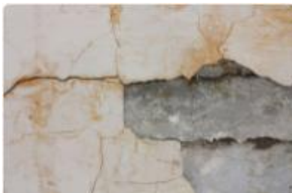
Figure IX .6 : alkali-réaction
