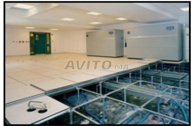
Figure (35): planchers technique
