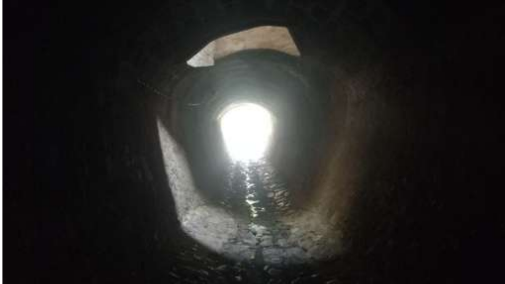
Photo 5-5: Tunnel existant au PK0+600.
