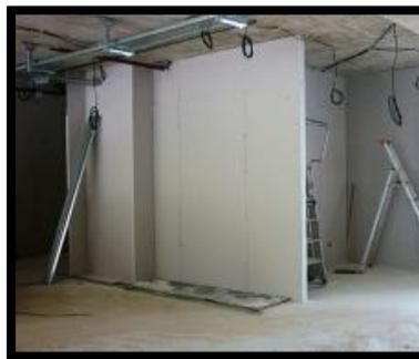
Figure 108. Cloison placoplâtre
