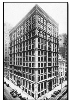
Figure 05 : Home insurance building
