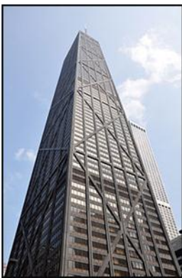
Figure 79 : John Hancock Center
