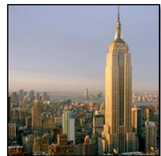
Figure 11: L'empire State Building
