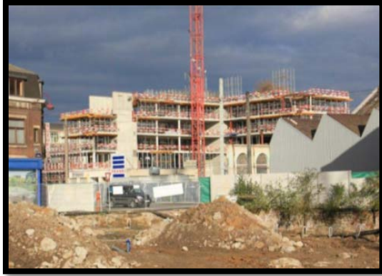
Figure 39 Centre CIM chantier
