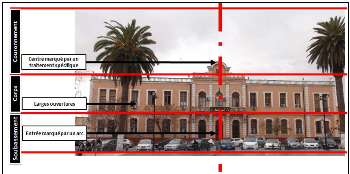
Figure 88 Façade principale tribunal
