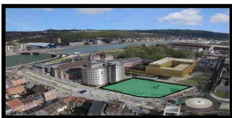
Figure 47 L'esplanade Kuborn –chantier-
