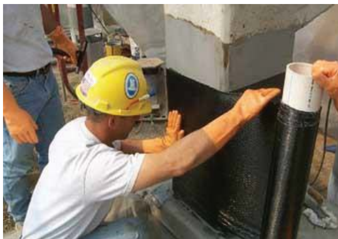
(a) Renforcement d'un poteau [3]
