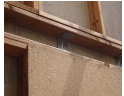
Figure 126: mur ossature bois en rideau
