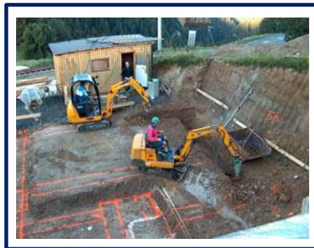
Figure 113: Terrassement (Source : www.Terrassement.com )
