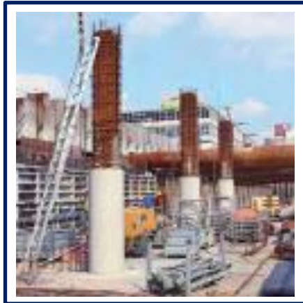
Figure 121: Coulage Poteaux mixte 25
