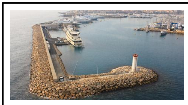
Figure 145: digue de protection maritime (Source: www. Digue de protection maritime.com )
